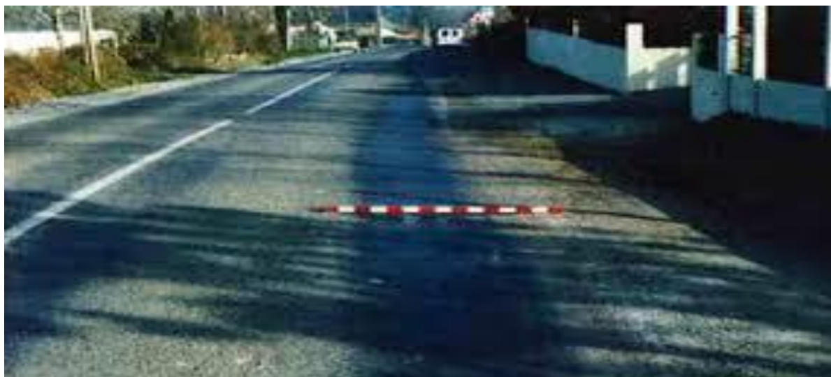
Figure 10 Glaçage [3]
