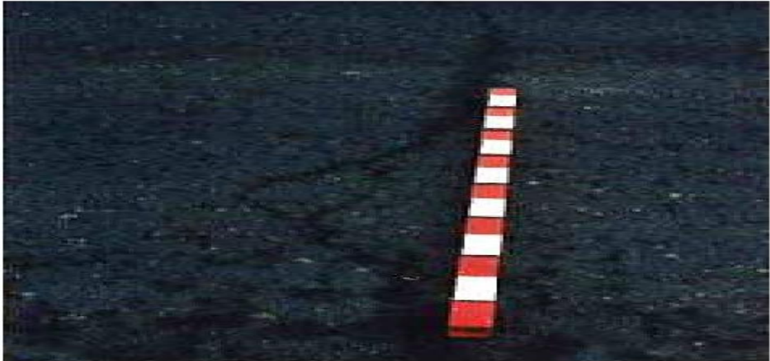
Figure 12 Fissure transversale [3]
