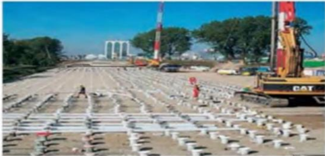
Figure I.23. Principe Installation des drains. [3]
