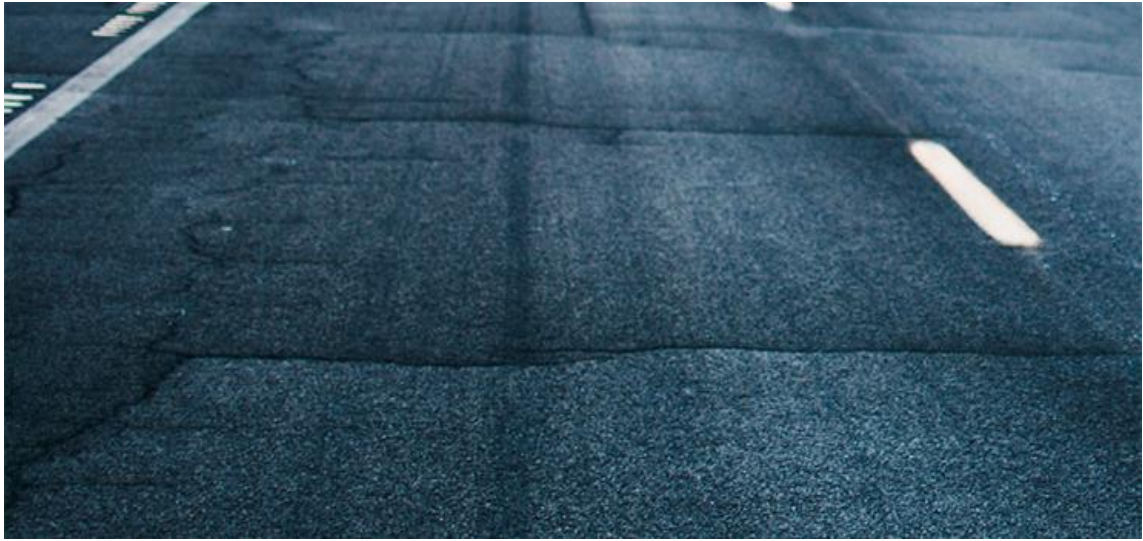
Figure 2.1. Fissures transversales
