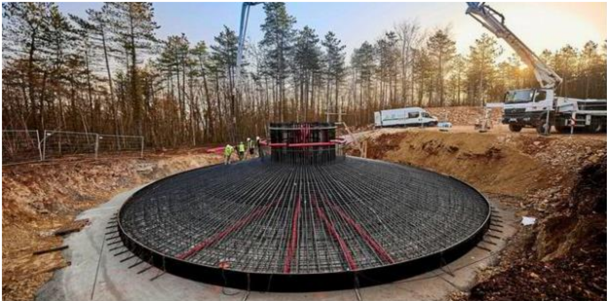
Figure I.3 classic onshore wind turbine foundations [62]
