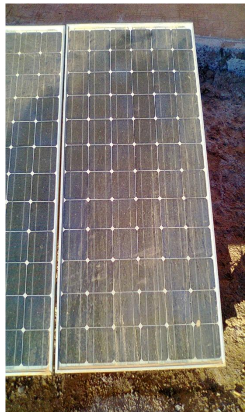
Fig.10. Dust accumulation on PV modules surface.
