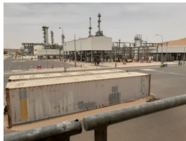
A.8: Central Processing Facility (CPF)
