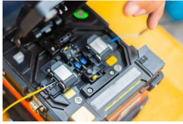
A.1: Fiber Optic Cables and Splicing Work
