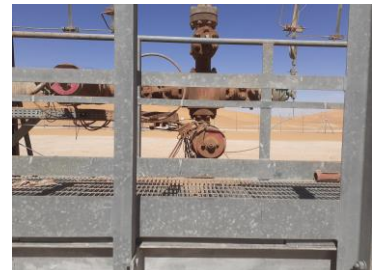
A.9: Oil Well Site
