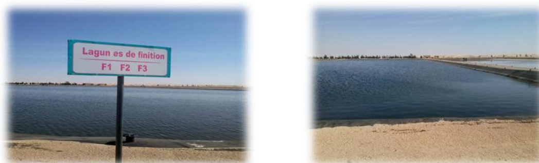
Figure 25: Lagune de finition.
