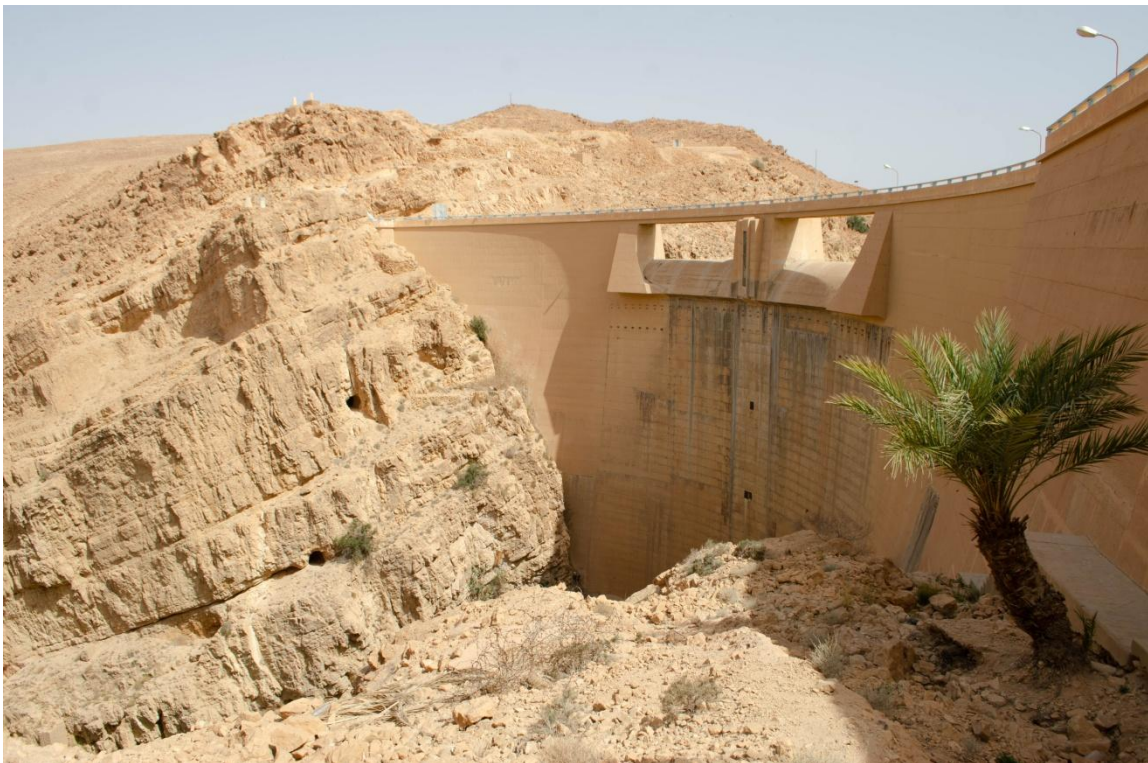
Figure II.2. barrage de Foug El Gherza (mai 2022)
