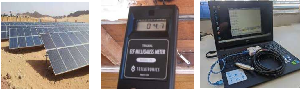
Figure III.7: SOLO LINE LX-100M photovoltaic panel installed at URAER with data acquisition instruments.
