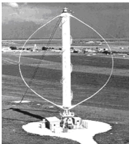
Figure II.4 : Exemples des constructions VAWT
