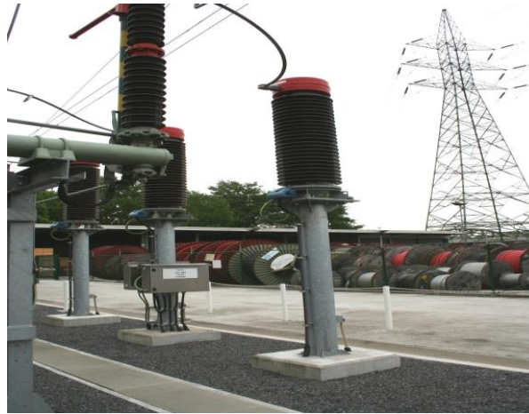
Figure III.3-Transformateur de tension.
