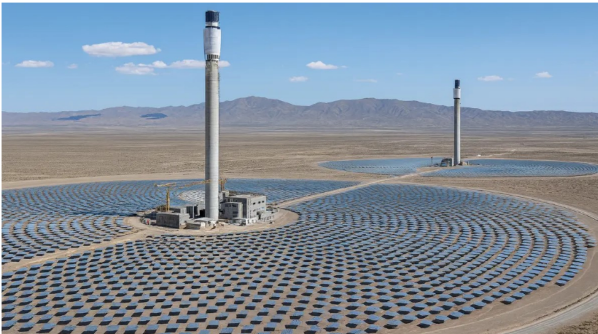
Figure I.9: Solar power towers
