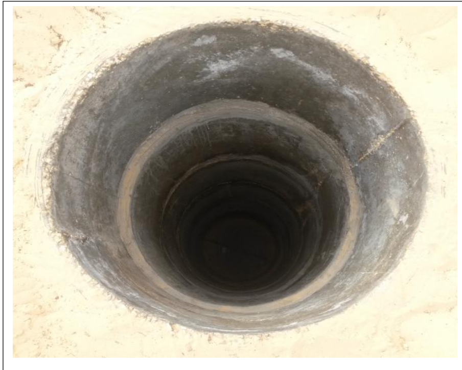
Fig (III.2): picture of the drilled well
