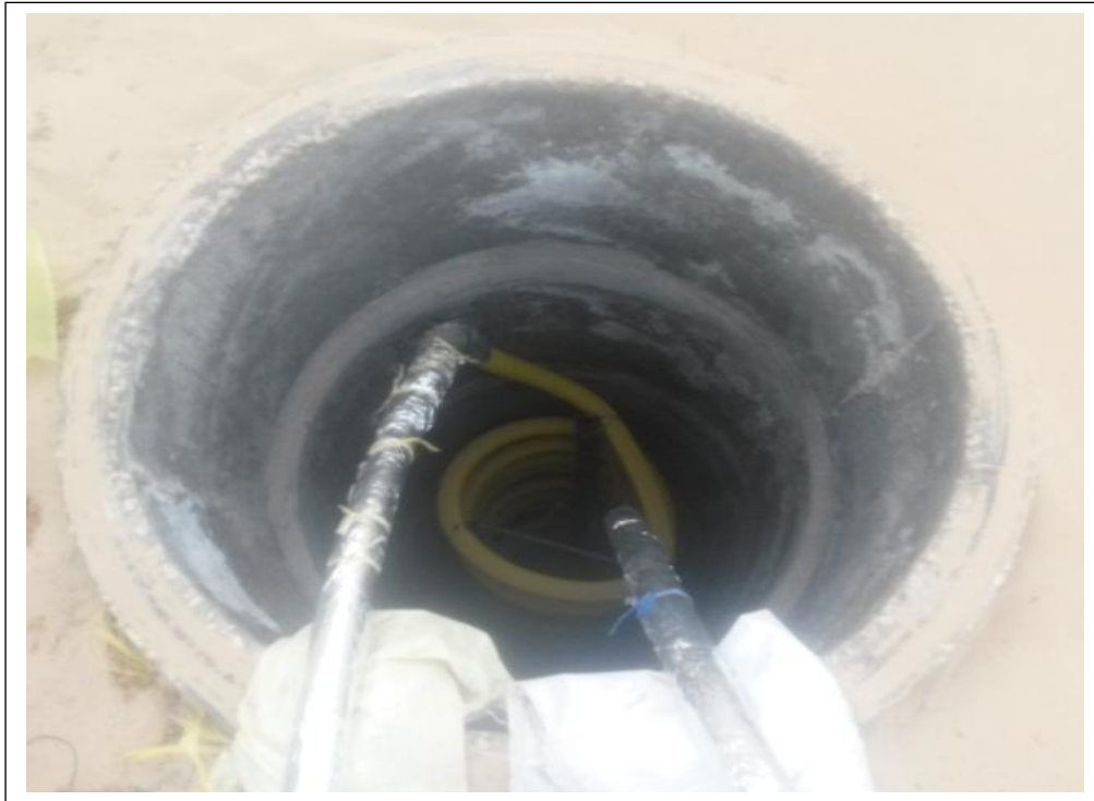
Fig (III.4): Setting up of the heat exchanger
