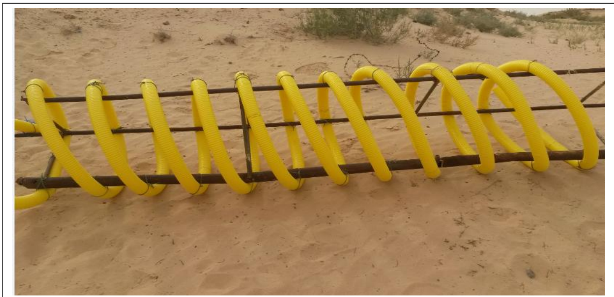
Fig (III.3): preparation of the exchanger
