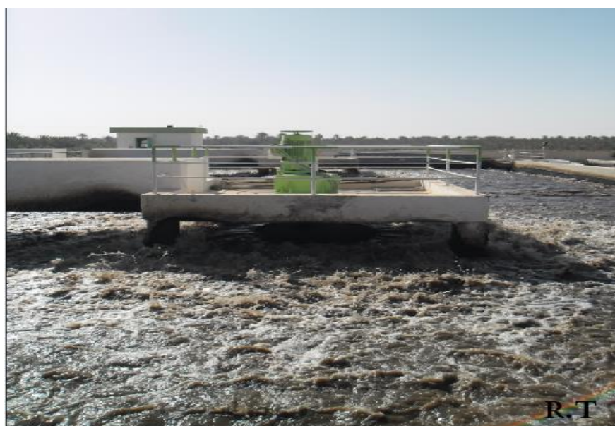
Photo 4: Bassin d aeration.
