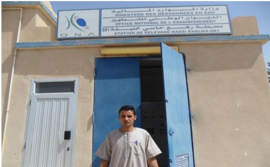
PHOTO II.8 : Station de relevage SR 01.
