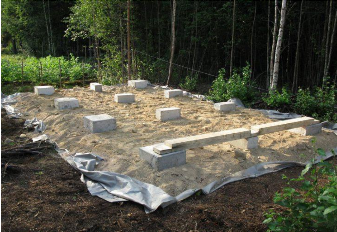
Figure I.9. Preparing the foundation
