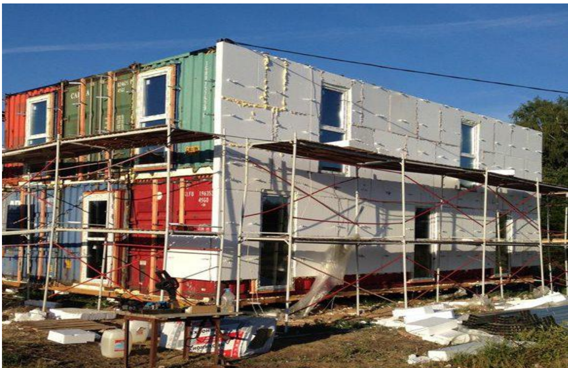
Figure I.11. Example of wall insulation with foam plasti
