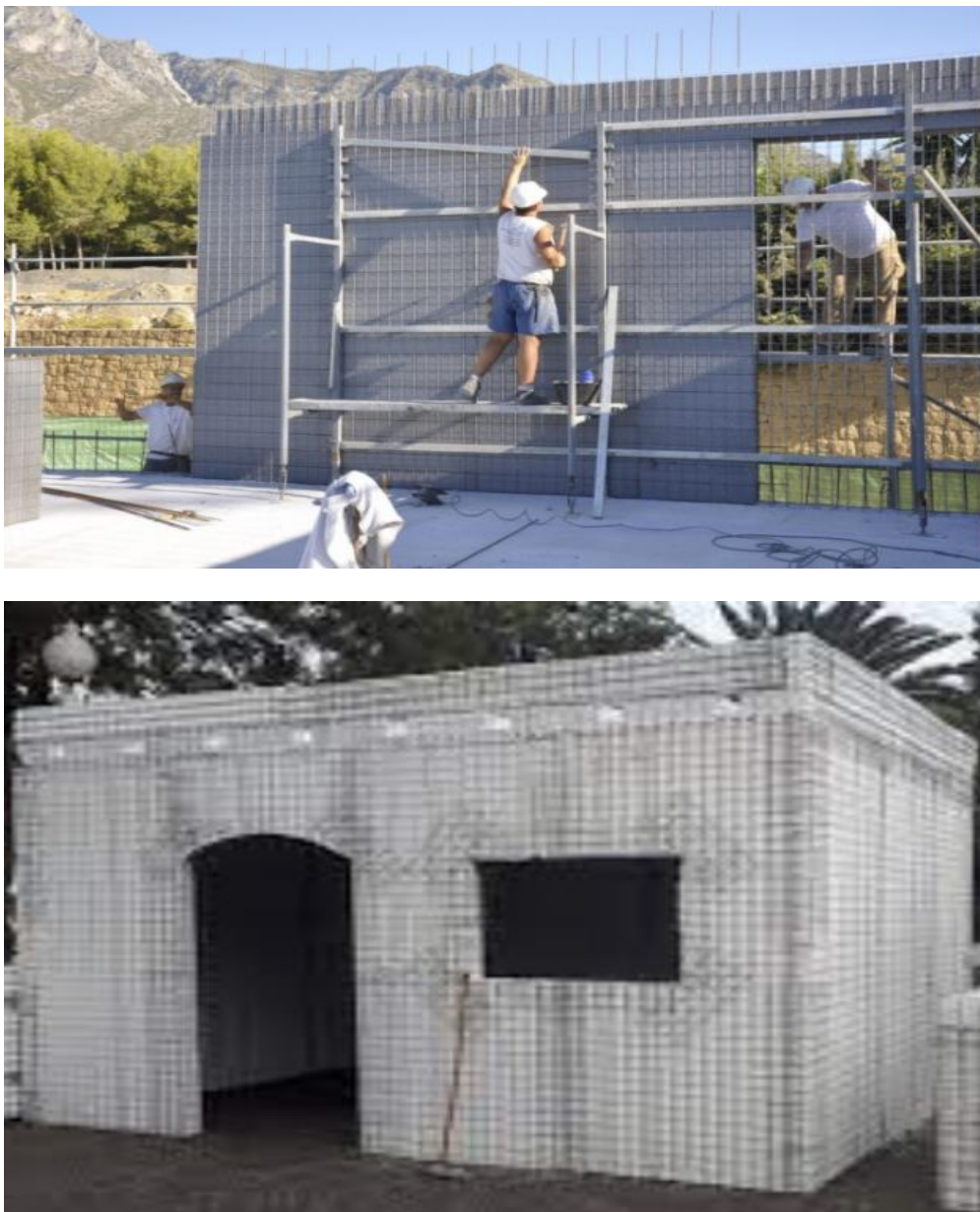
Figure I.17. Stages of building a Polystyrene house
