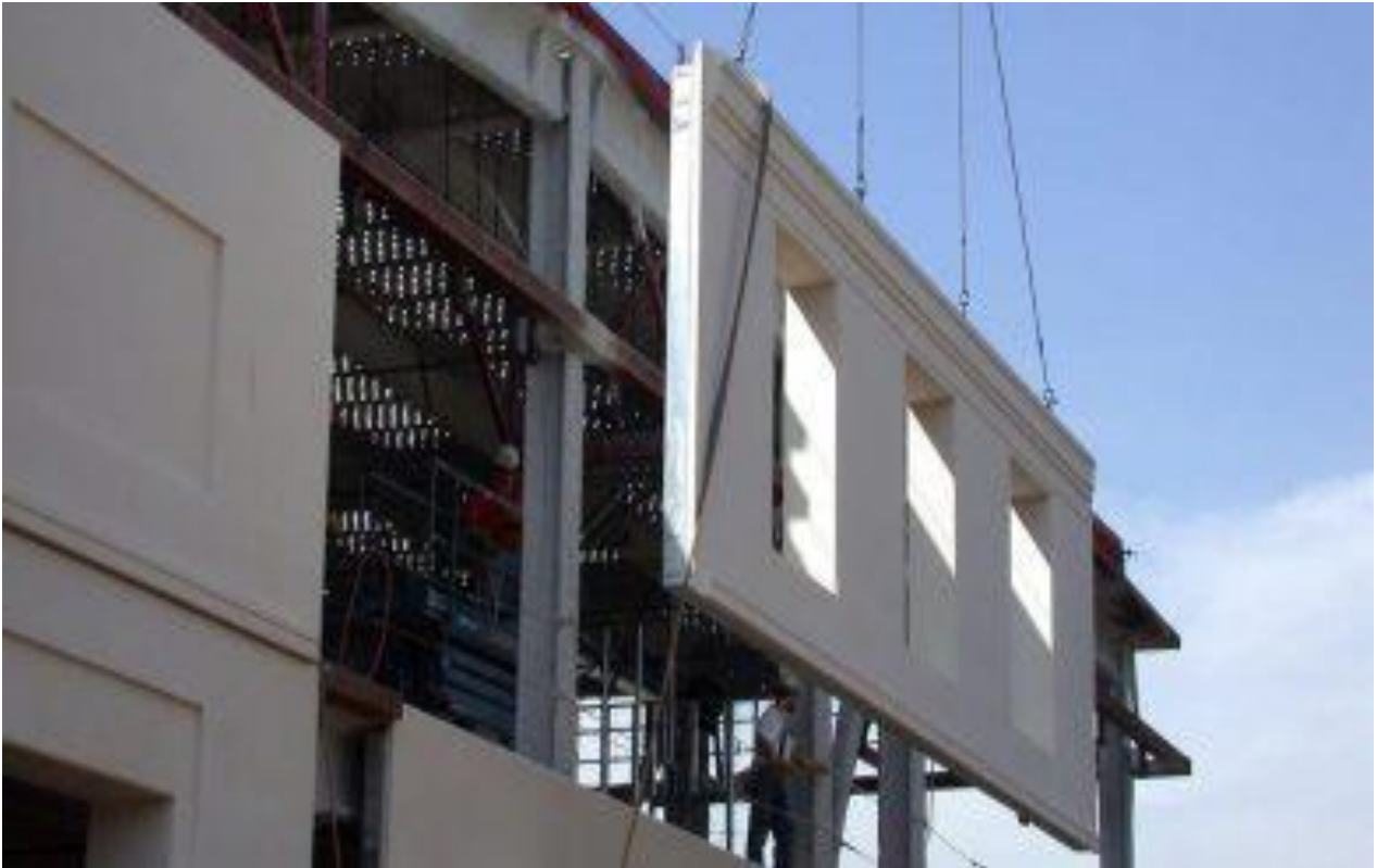
Figure I.16. Installation of precast concrete walls
