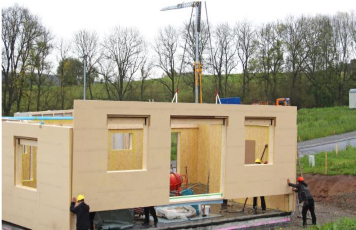
Figure I.14. Assembling a prefabricated wooden house
