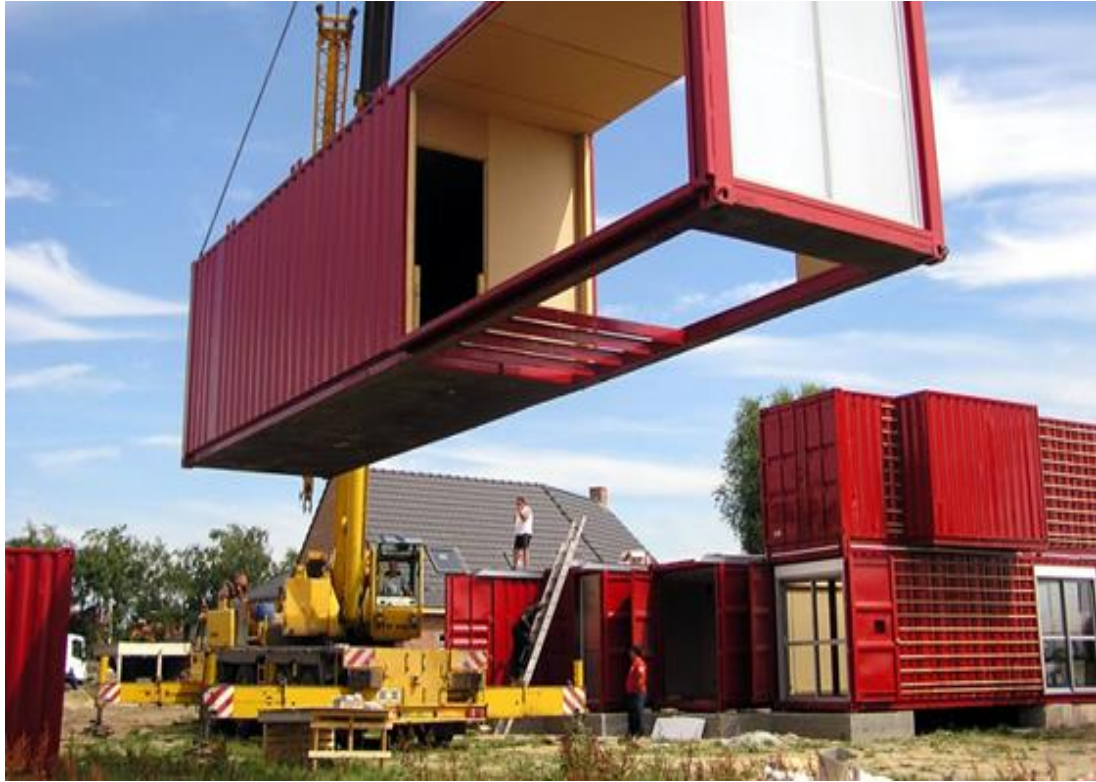
Figure I.10. Container installation
