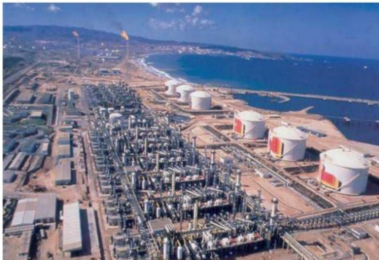
Figure II.5 : station raffinerie des Arzew [29]
