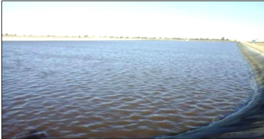
Figure 15 : Lagunes de finition (ONA, 2019)
