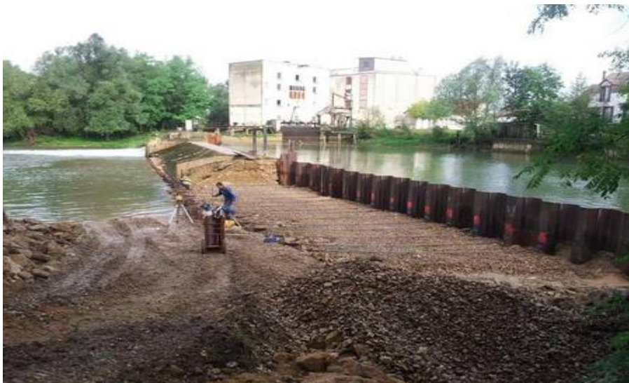
Figure 6. 1. Barrage de consolidation.
