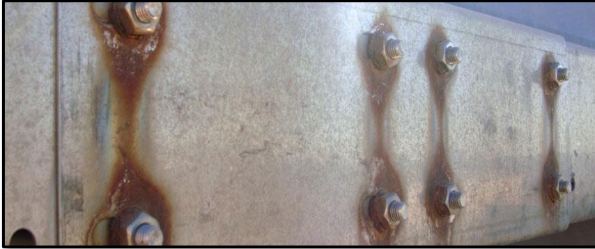
Figure III.2 corrosion galvanique
