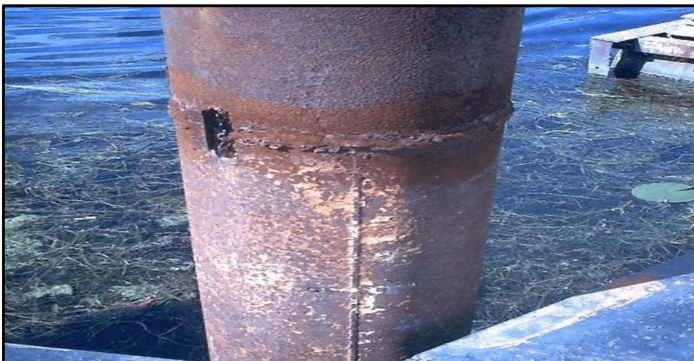
Figure III.1 corrosion uniforme
