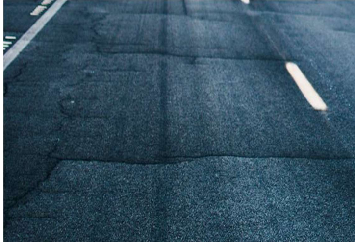
Figure 2.5. Fissures transversales
