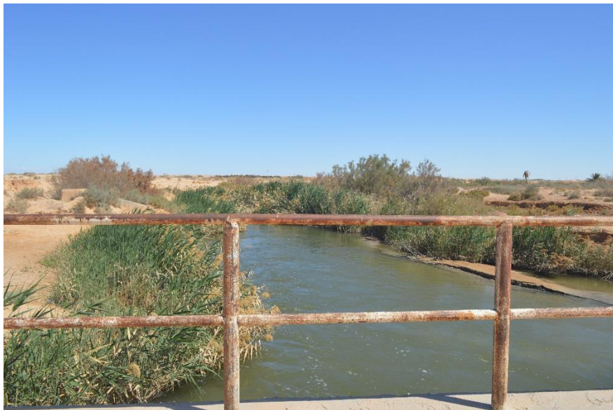
Photo III-5 canal principal de la station boufeggoussa
