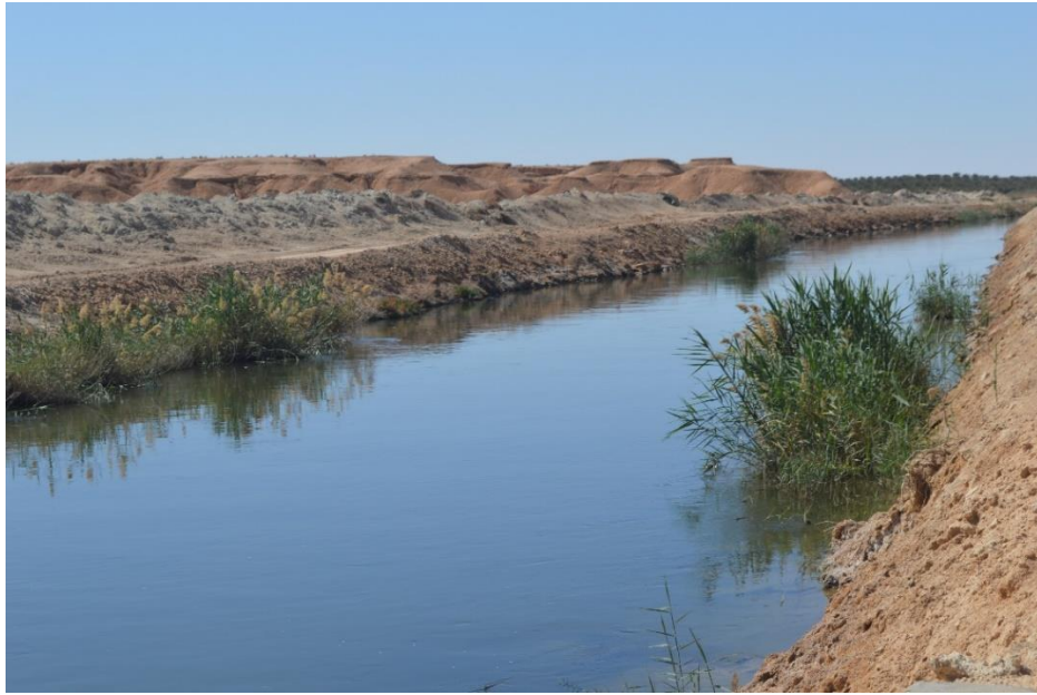
Photo III-4 canal principal du station Tendla Aval
