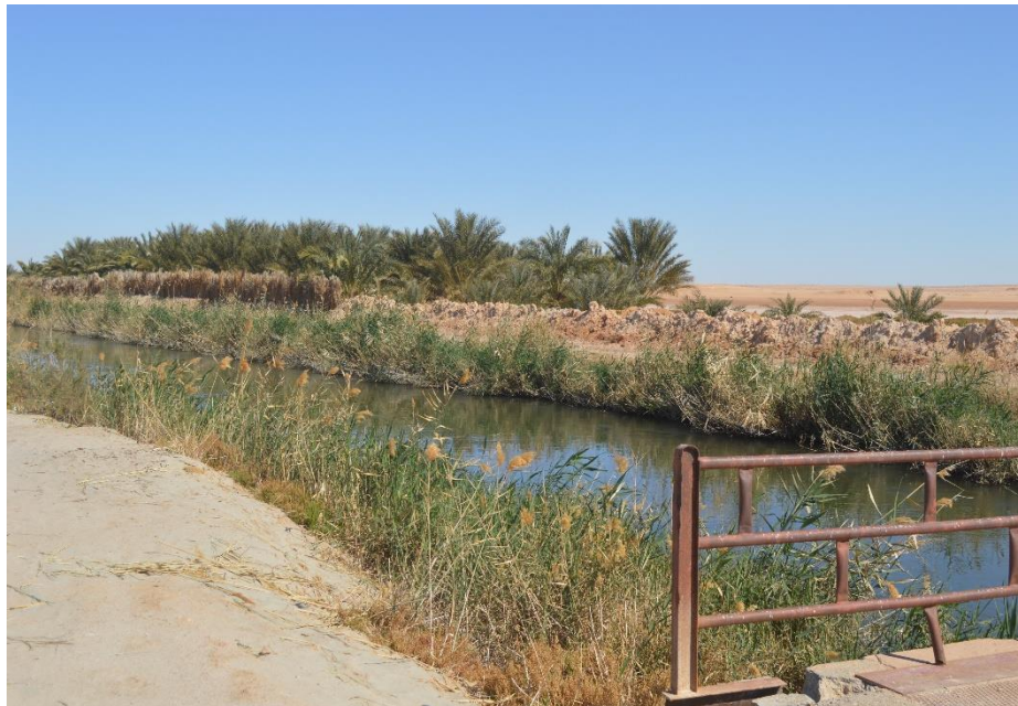
Photo III-3 canal principal du station Tendla Amont
