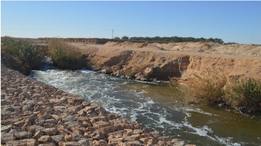
Photo III-1 canal principal du station S. amrane
