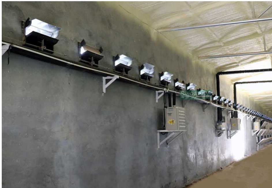
Figure 16. Poultry sidewall inlets - wall vent poultry house ventilation [45].
