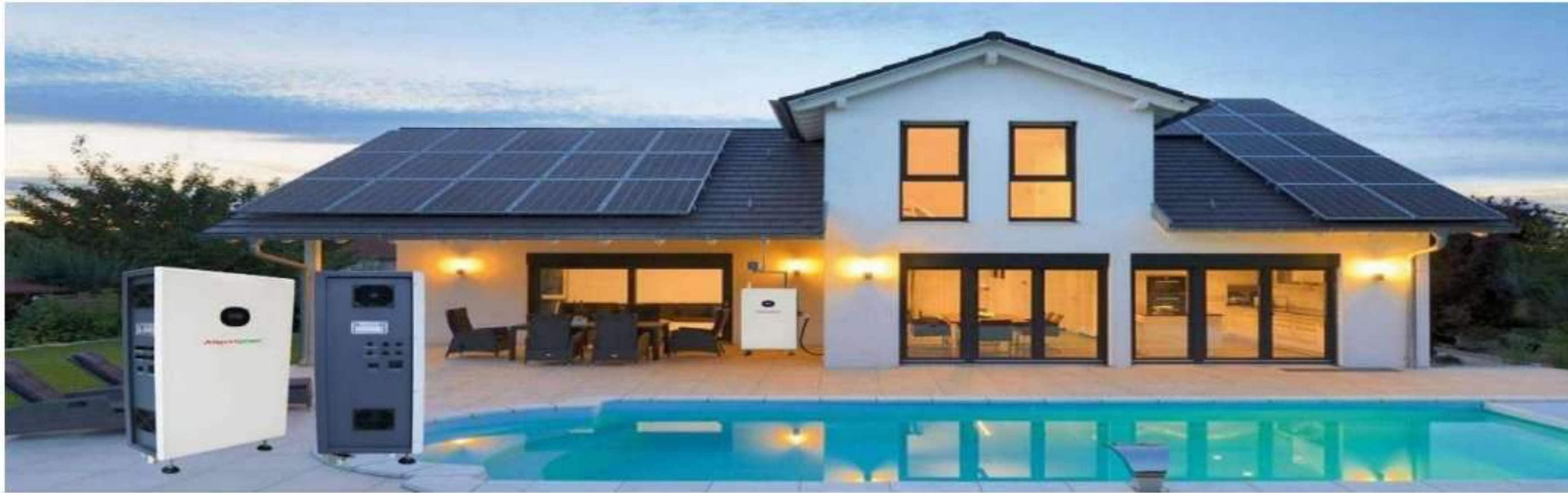
Figure (1-13): Home battery storage
