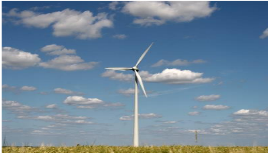
Figure I.9. Horizontal axis wind turbine.
