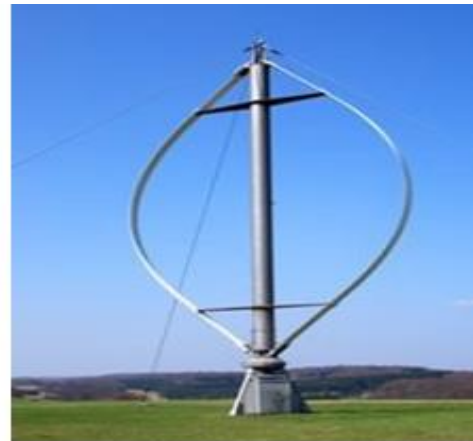
Figure I.12: Darrieus-type wind turbine
