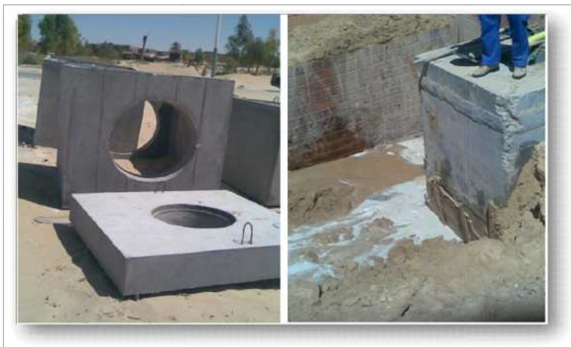
Figure V.5: Construction des ouvrages surplace
