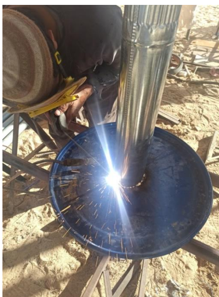
Photo03: Welding the tube in the lid to simulate the chimney.
