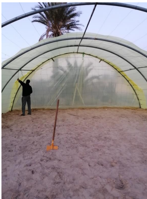
Photo09: The greenhouse preparation
