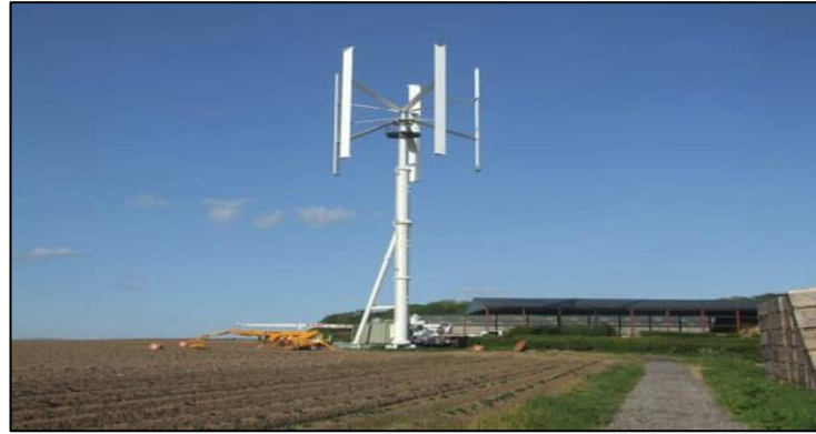
Figure I. 13 Giro mill wind turbine
