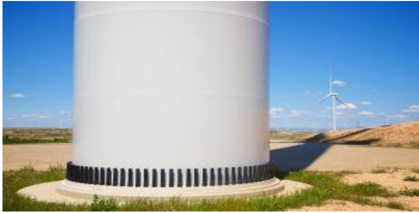
Figure I. 3 turbine Wind foundation
