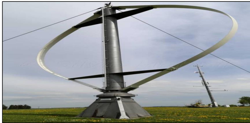
Figure I. 11 Darrieus turbine by guy-wire.
