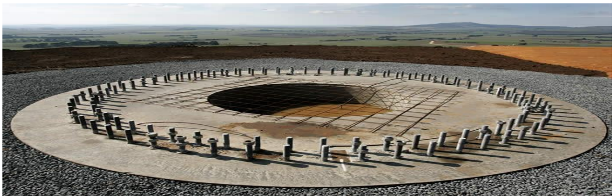
Figure.II.4. Concrete foundation of onshore wind turbine.
