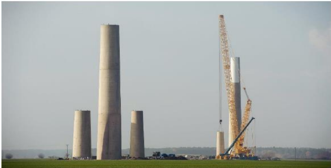
Figure.II.8. Concrete towers for wind turbines.
