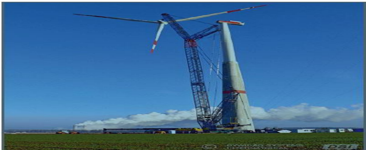
Figure.II.9. Assembly process for hybrid tower.
